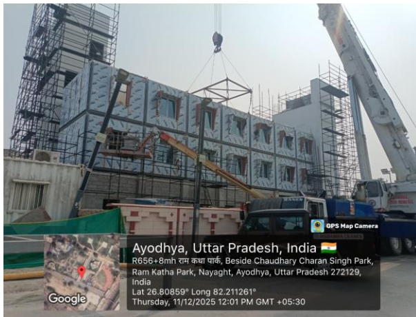
Construction at L&T PPVC Site
